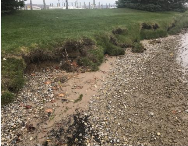
Eroded shoreline property with no greenbelt present.
